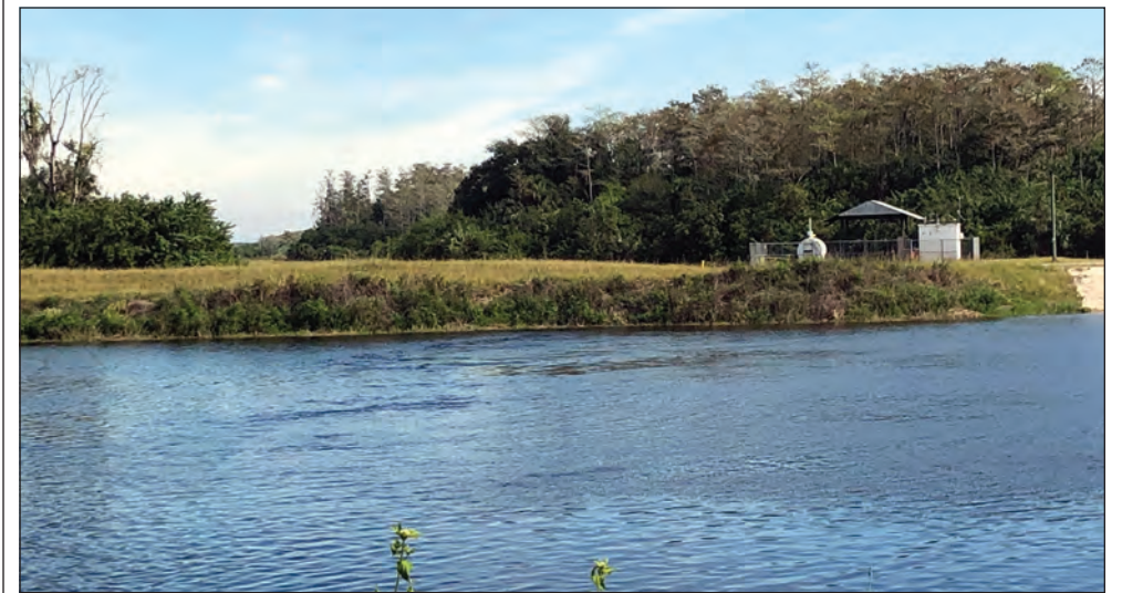
Courtesy photo The E2 pump in Big Cypress feeds water into the north feeder by the S190 structure.
