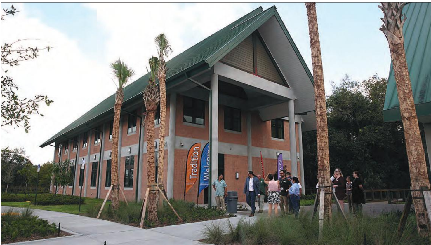
The Major Billy L. Cypress Building, which houses the THPO department and Ah-Tah-Thi-Ki Museum employees, opened in Big Cypress Oct. 23.
