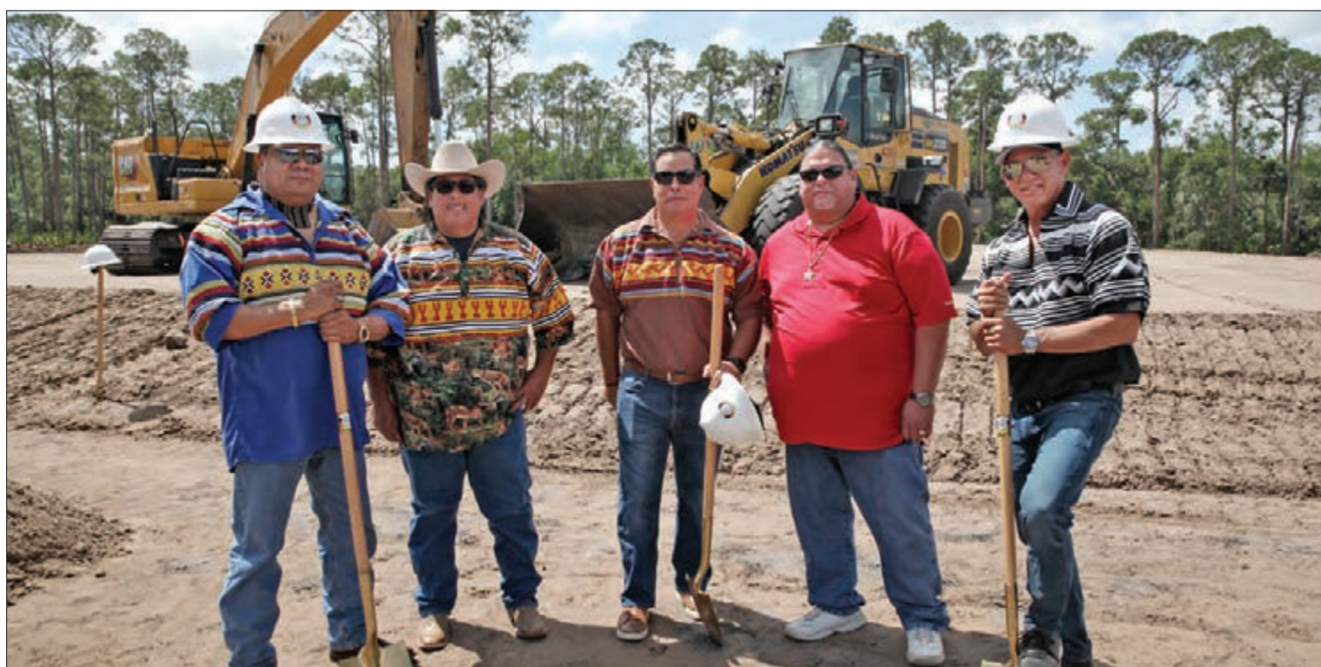
From left, Brighton Councilman Larry Howard, Immokalee Council liaison Ray Garza, Chairman Marcellus W. Osceola Jr., Immokalee Board liaison Ralph Sanchez and Hollywood Councilman Chris Osceola at the Immokalee construction site after the official groundbreaking. Beverly Bidney
