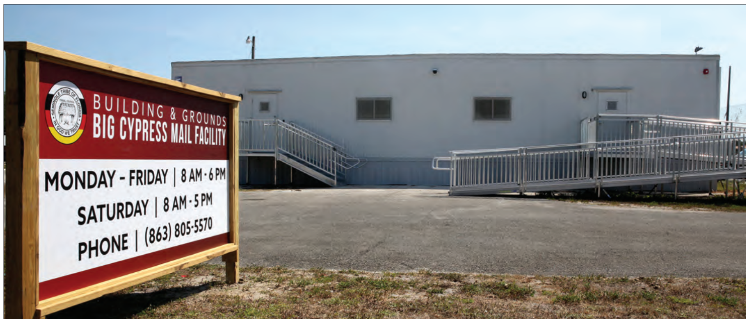
MAIL CALL: A new mail facility recently opened in Big Cypress at 30550 Josie Billie Highway.
